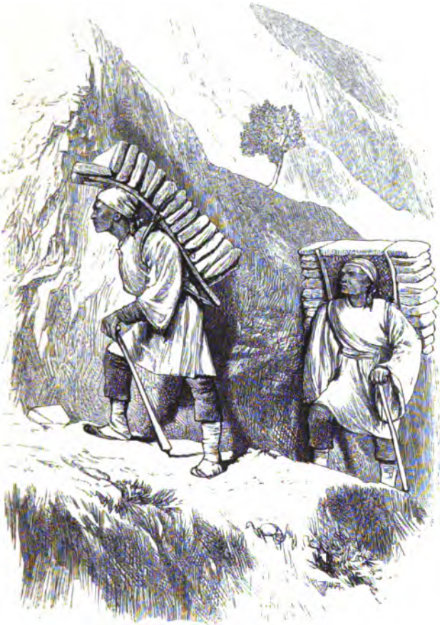
COOLIES CARRYING BRICK TEA.
